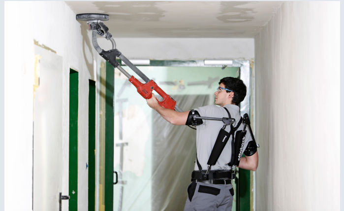
Figure 16: The Paexo Shoulder from Ottobock for working in construction
